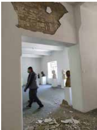
4. Pukotine na zidovima i stropovima u stalnim postavima. (Fototeka Gliptoteke HAZU) Cracks in walls and ceilings in permanent exhibition spaces. (HAZU Glyptothèque photo files)
