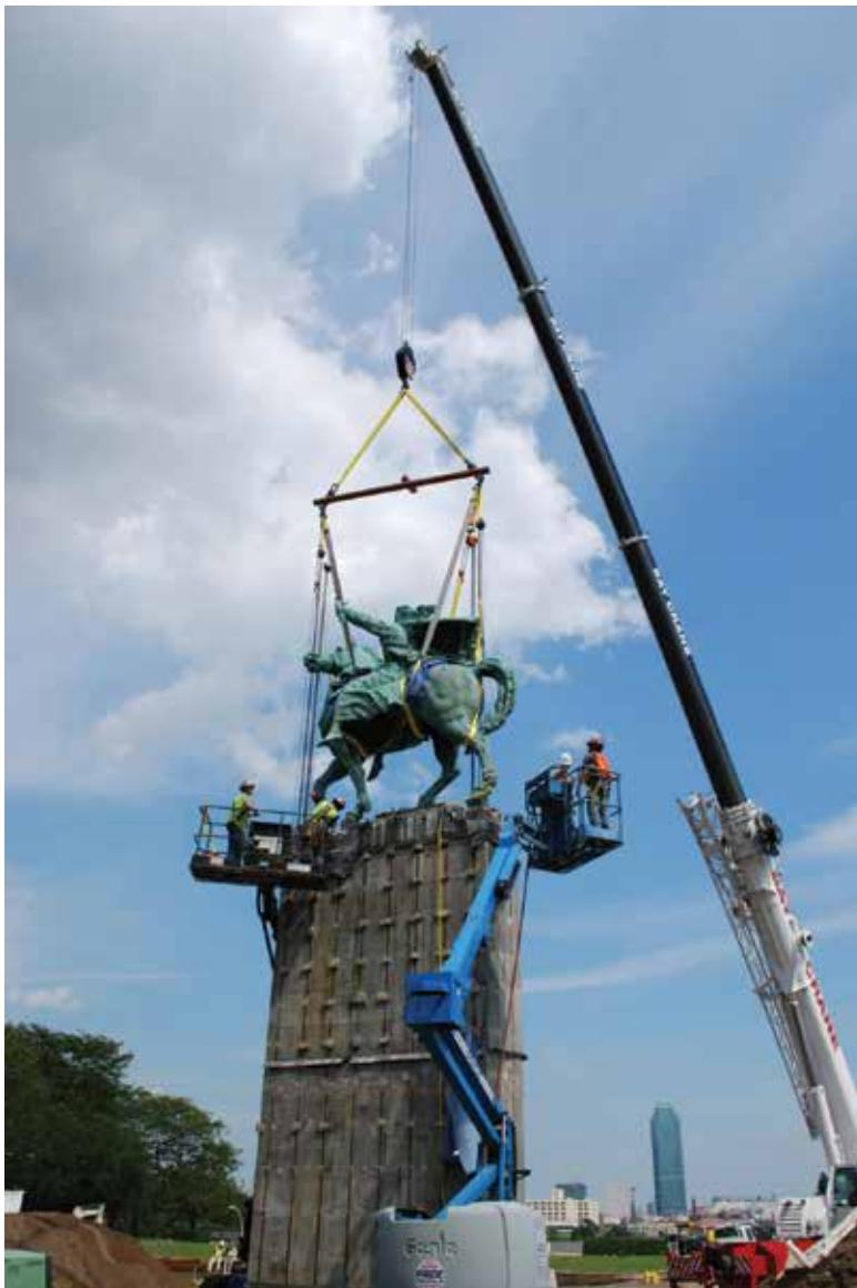
Rigging Operations for De-Installation 2008
