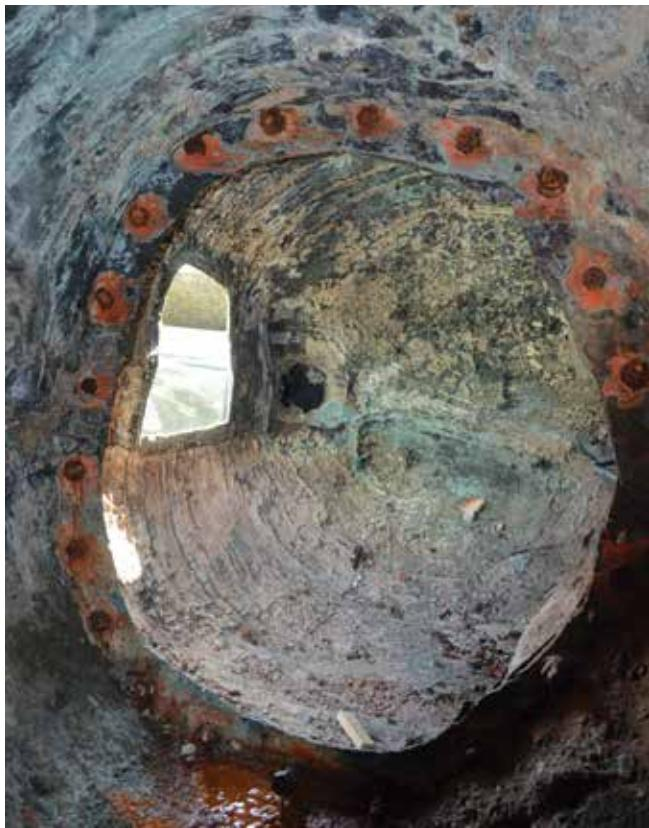
Interior Original Bolted Connections Mid-Section of Horse
