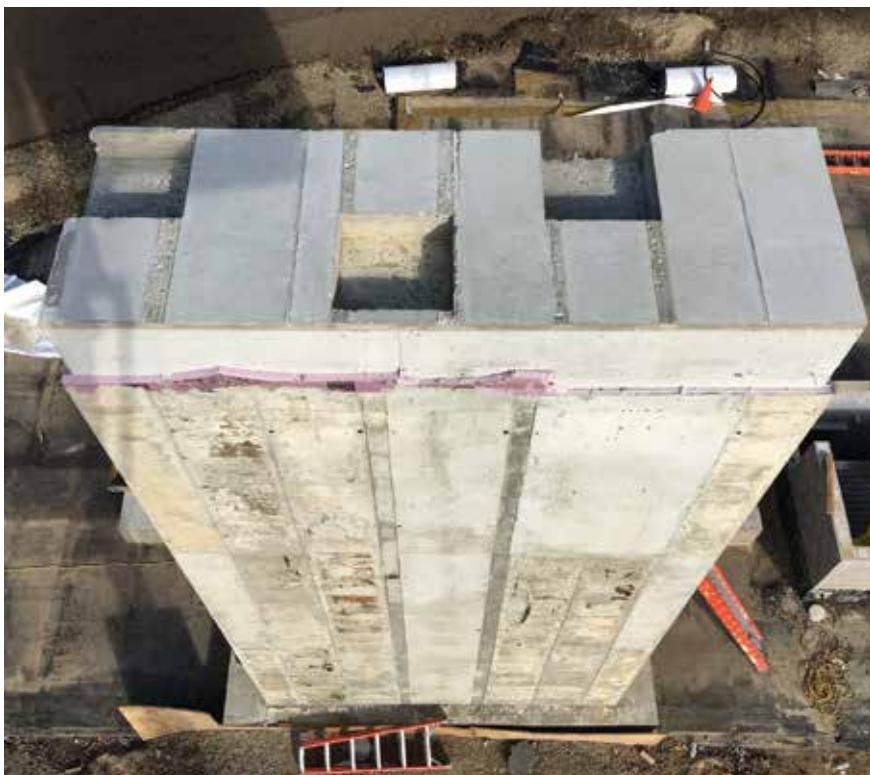
Cement Pedestal with Cut-Outs for Mounting
