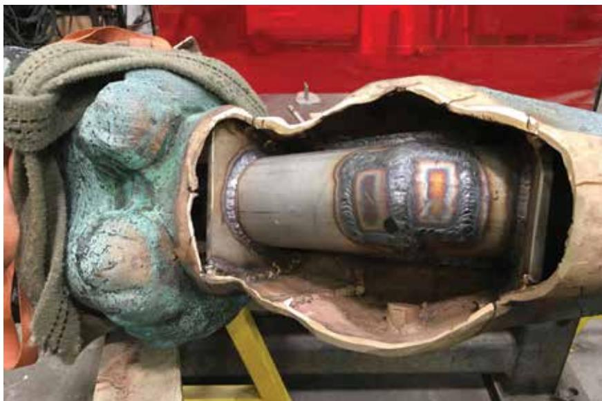
Installation of Pipe at Fetlock with Gusset Plates
